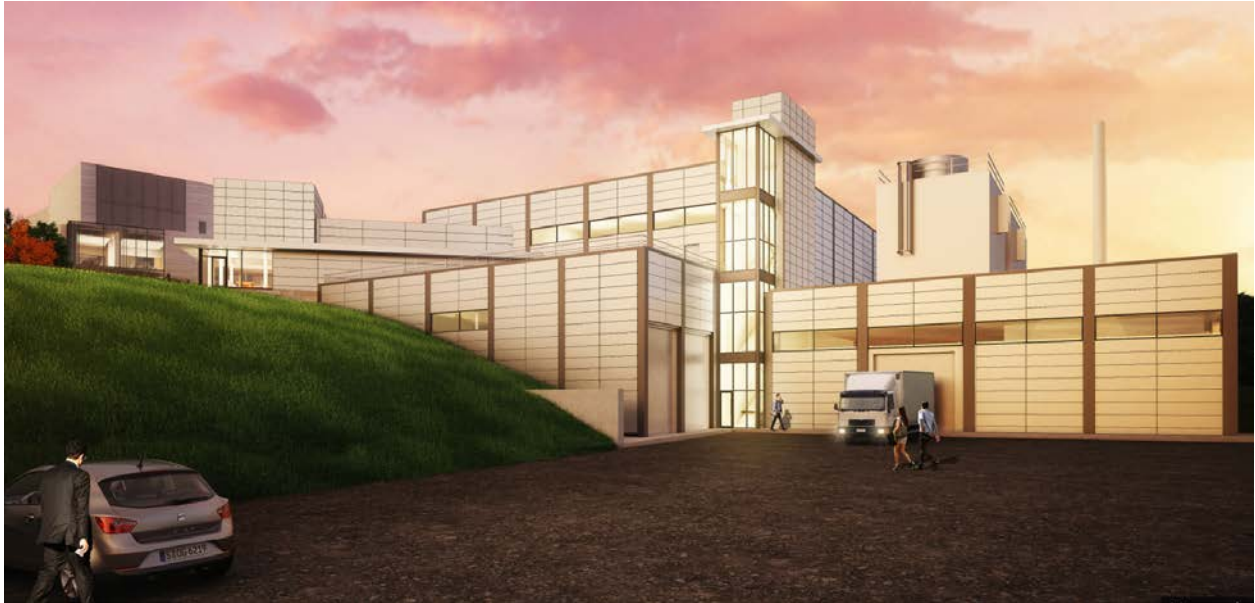
Supplemental Utility Plant lower level – from King Hill Road
