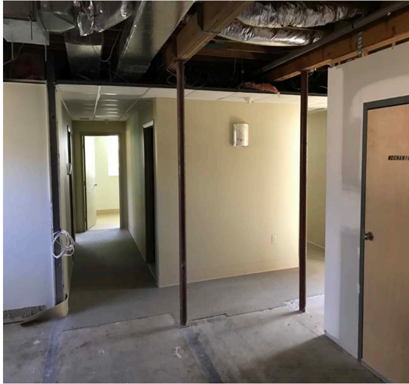
28 Professional Park – Interior Space
